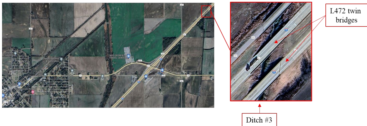
Figure 2.12 Satellite images of the L472 Bridge site
