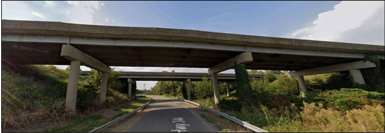
Figure 2.5 A1466 Twin Bridges (real image)
